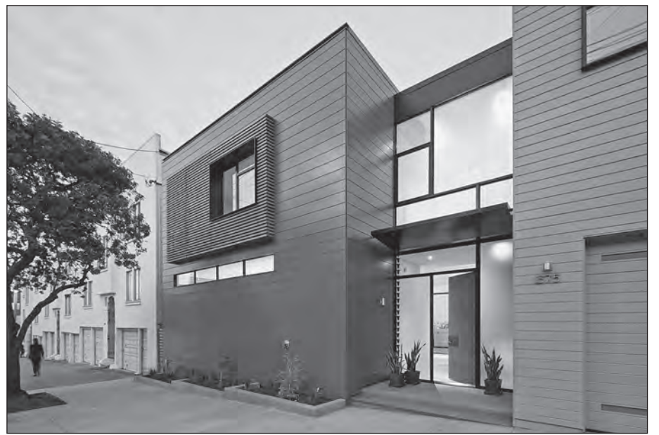
This modern showcase on Noe Street, designed by San Francisco’s Studio VARA, will be a stop along the Sept. 20 home tour hosted by AIA San Francisco as part of the “Architecture and the City Festival.”
